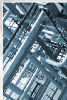
Heating equipment inspection
